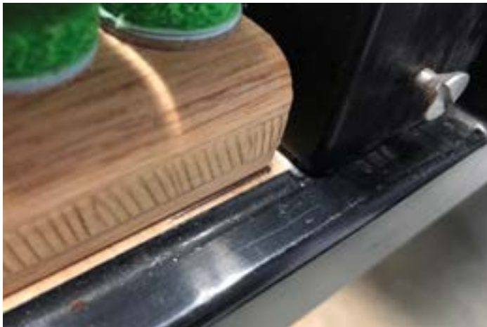
The front rail position marked on the keybed with a pen.
