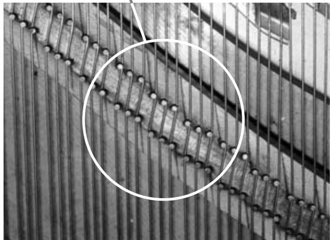
**Figure 109** This style of notching in a ca. 1900 New York Steinway concert grand model D creates unequal speaking lengths of strings in unisons in the mid-treble section. The purpose of unequal speaking lengths is to improve sustain in the “melody” octave.
